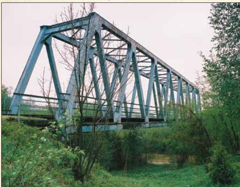
Brzeźnica - Most / Steel railway bridge
